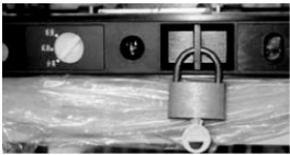
抽屉式断路器 “分离”位置锁定挂锁器 "Seperated" position locked with padlock for draw-out breakers
