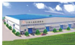
现代化生产车间 Modern Production Workshop
