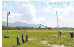
Provincial power grid of Rural upgrades and renovation
