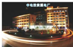
CLP Guixi power plant
